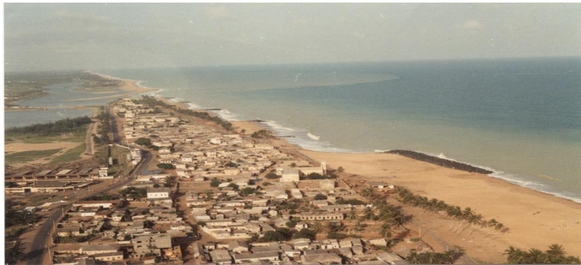
Figure 5. Coastal protection measures in Togo.
