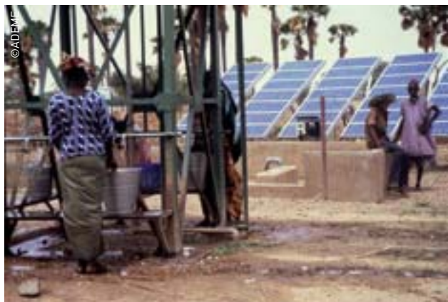
Solar for water pumping
